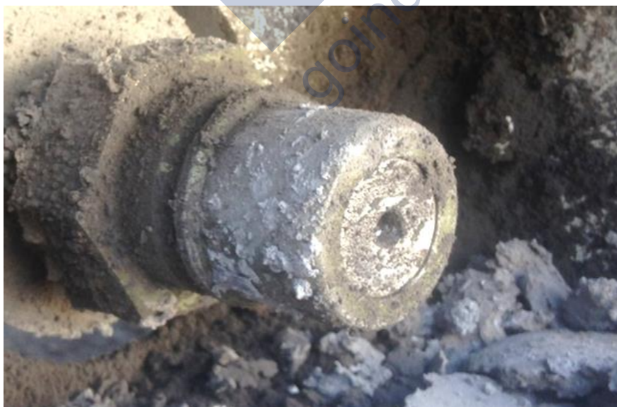
Figure 25 - Contaminated Receiver - No Dust Cap Fitted
