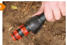
Position the in the body of fitting, positii the grip ring nut and tight hand.
