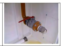
80nb Overfill Protection Valve c/w Float Assembly
