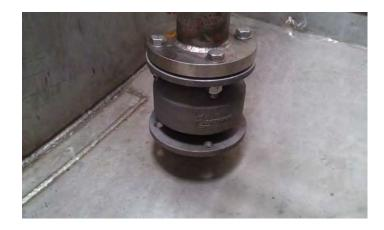
2. Foot Valve – the Anti Syphon Valve is designed and indeed positioned to also operate as a foot valve. The valve is designed to retain a full head of fuel on the dispensing equipment in order to provide an easy start for the next pumping operation. This is particularly important for centrifugal style pumps that do not provide self priming operation.
