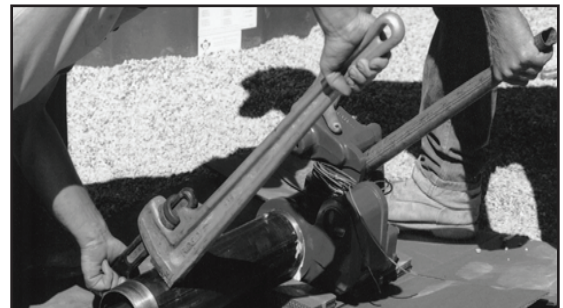
Figure 3: Attach Riser
