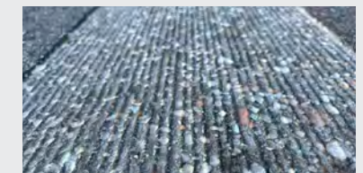
Creates coarse profile that's ideal for thick coatings and aggressive removal
